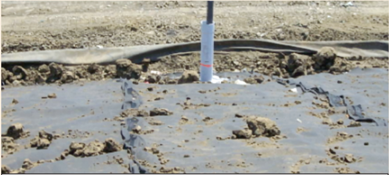
Photo 2. Geocomposite placed directly on waste interim cover—below final cover construction.
