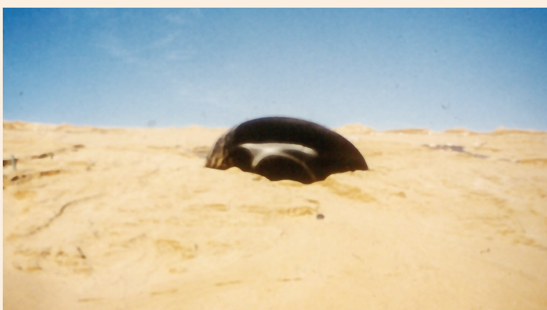
Photo 1. Geomembrane gas bubble during final cover construction.
