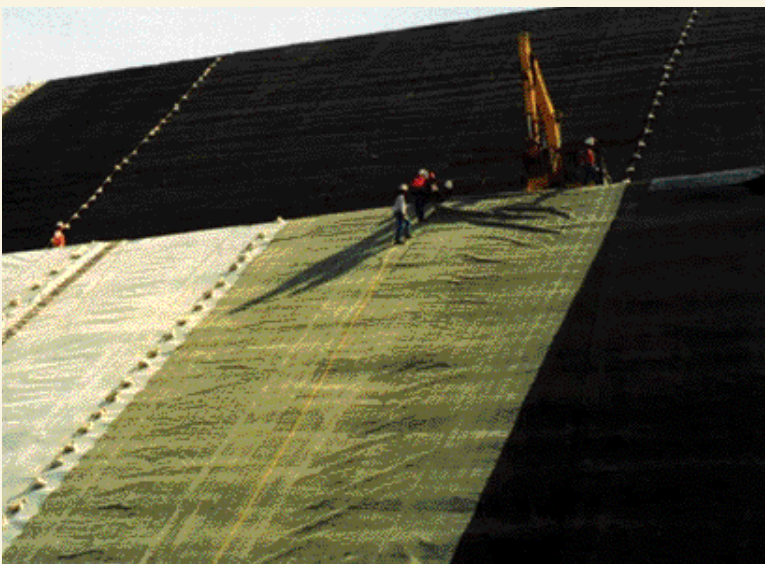
Photo 1: Installations of a GCL over a protective geotextile cushion.
