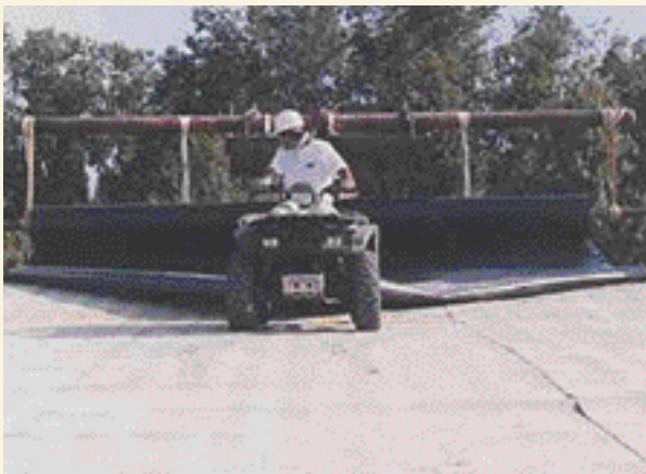
Photo 2: Deployment of a geomembrane over a GCL with an all-terrain vehicle.
